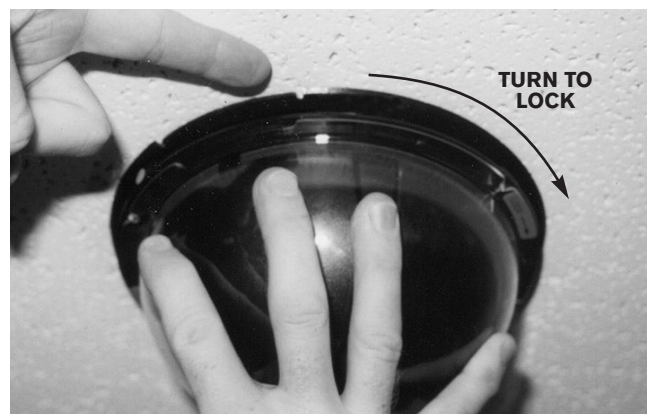
Photo 2G Lock dome into place
