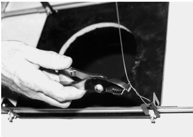
Figure 9.4: Fixation du support
