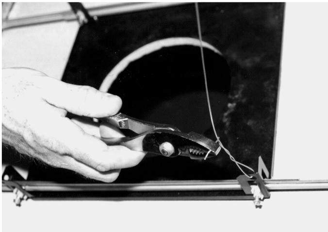
**Figure 9.4: Fixation du support**
